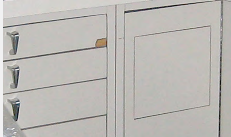
Custom cabinets are not made for the harsh operator environment. Over time they may warp, chip, and gap due to weakened door hinges.
